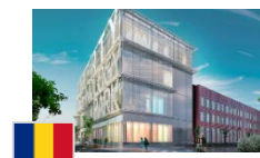
Liberty Technology Park, Cluj , Rumunsko
